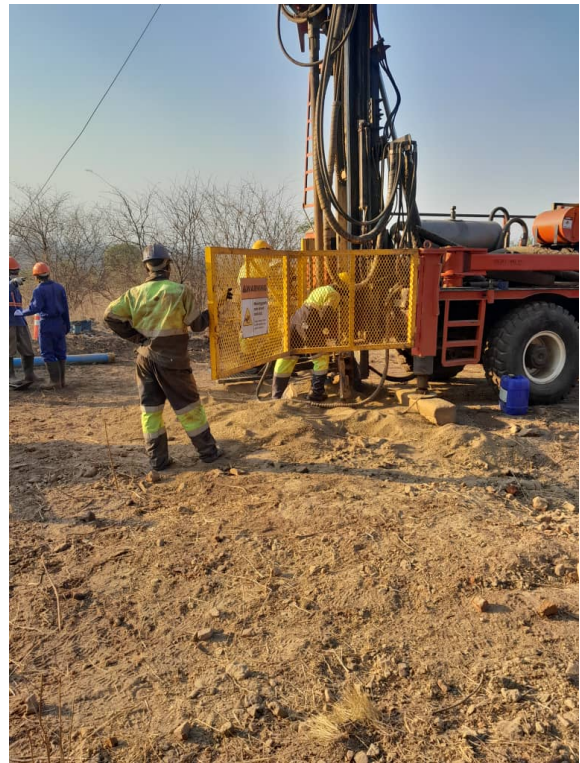
Drill hole preparation
