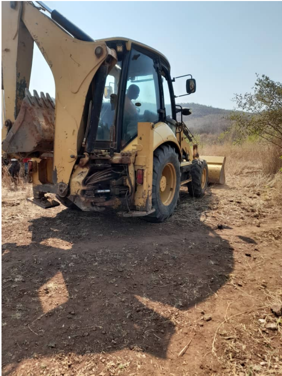
JCB onsite repairing hill top access roads
