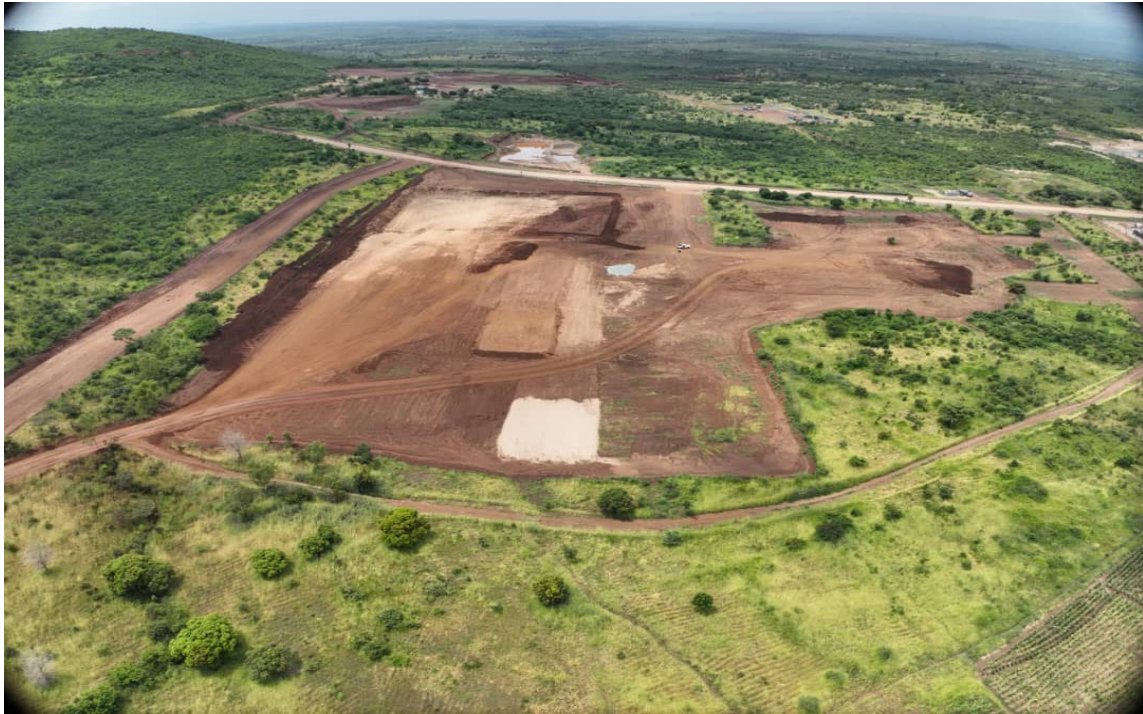
Figure 9: Mobile maintenance workshop precinct earthworks progressing, with the workshop platform and access routes being prepared to support fleet uptime and on-site maintenance during construction and early mining operations.
