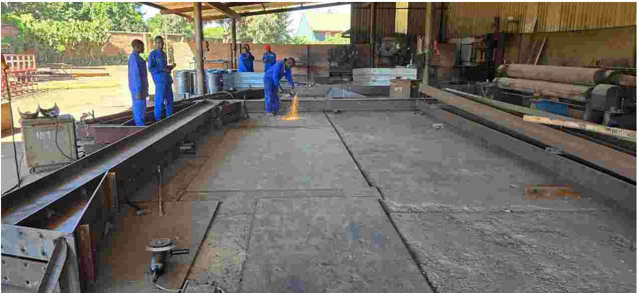
Picture 6. Offsite steel fabrication works
