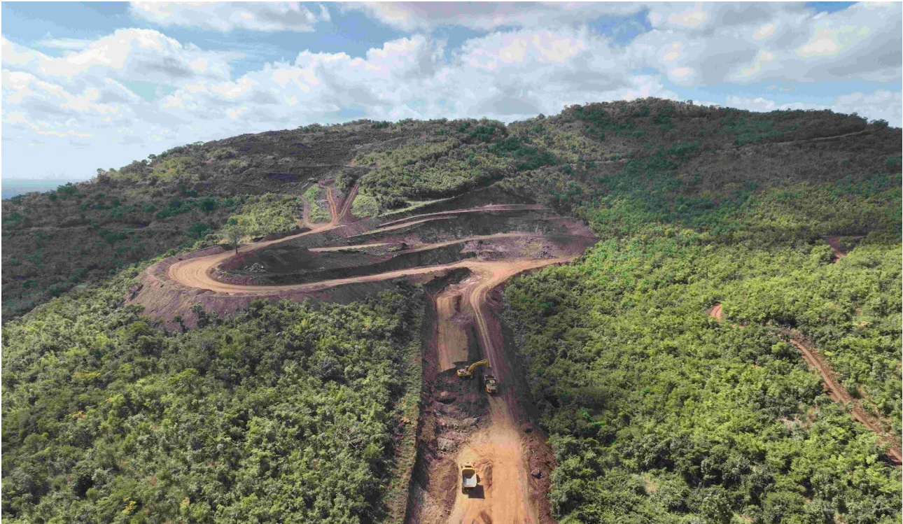
Picture 8. Haul road works at Kangankunde advancing
