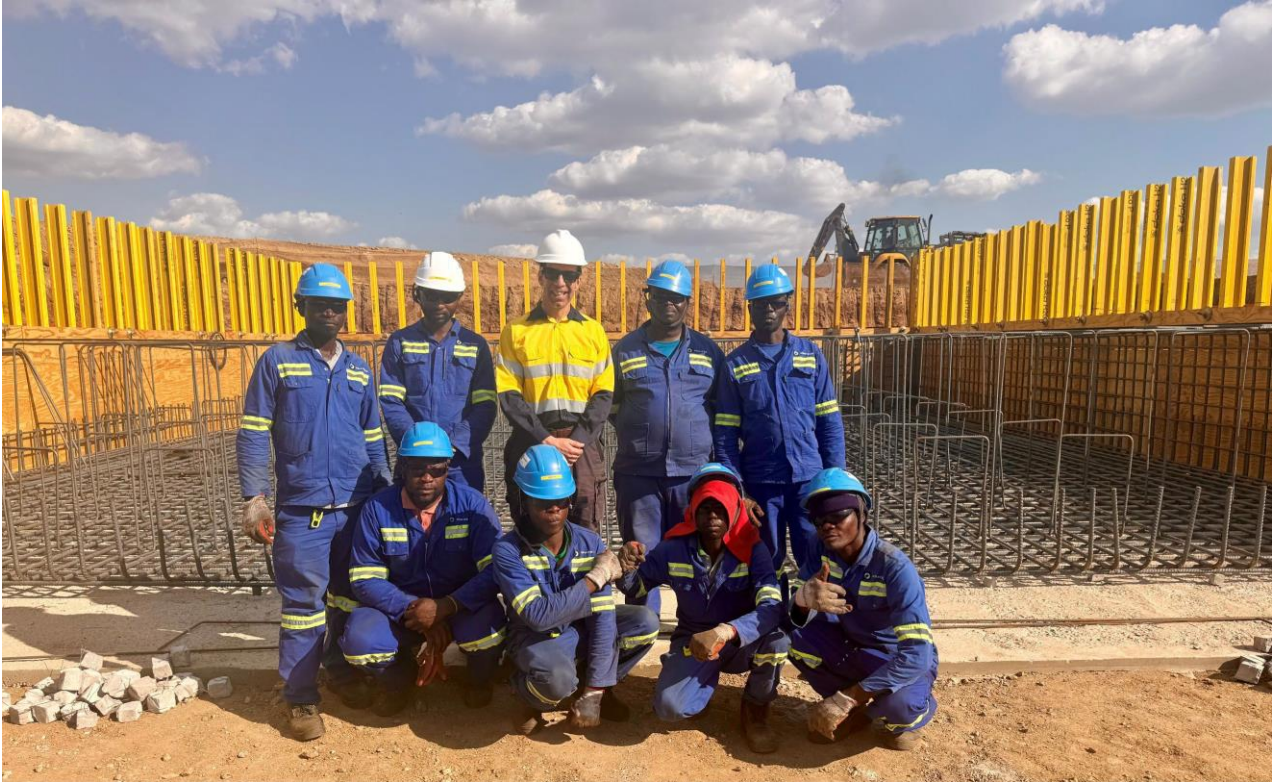
Picture 1. Lindian Resources Executive Director Zac Komur with the Kangankunde construction team at the SAG mill foundation area, where process plant civil works continue to advance
