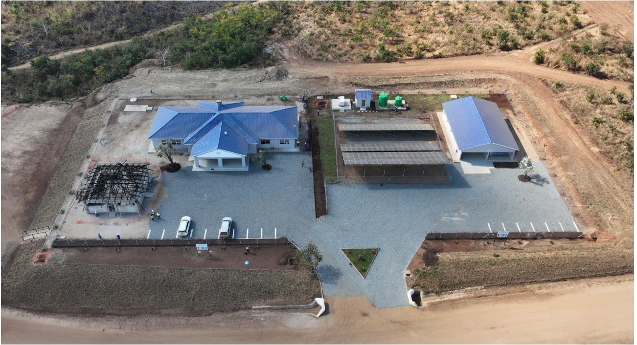
Picture 13. Kangankunde Administration and Medic Facility.
