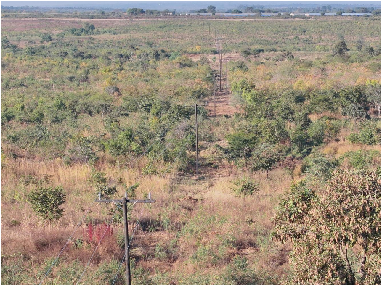
Picture 9. A section of the 27km power corridor
