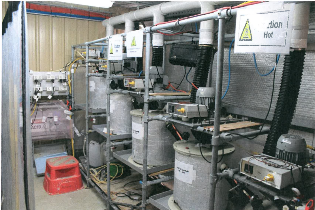
Figure 1 Spodumene pilot processing facilities at ANSTO Minerals, Lucas Heights, and Australia.
