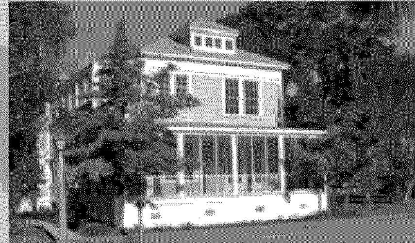
Completed Renovation of Historic Quarters #4
