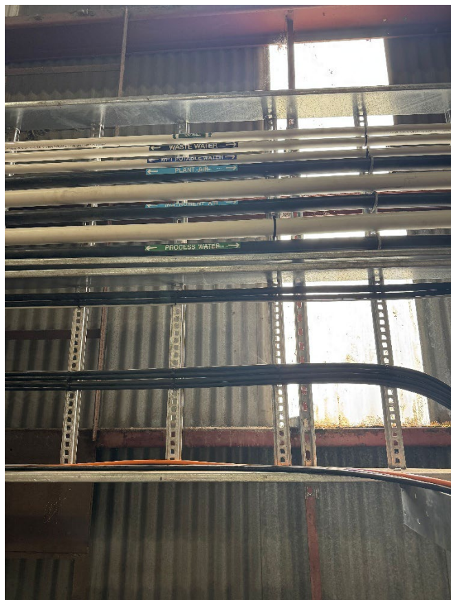
Exhaust stack support fabrication, utility piping, and argon supply installation complete
