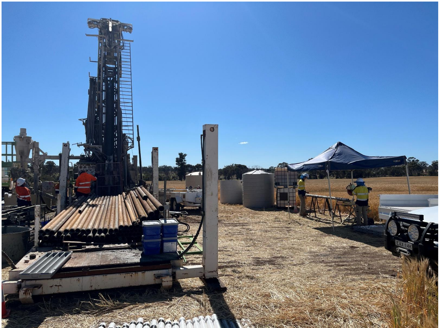
Figure 1: Drill Rig mobilised at the Dam deposit
