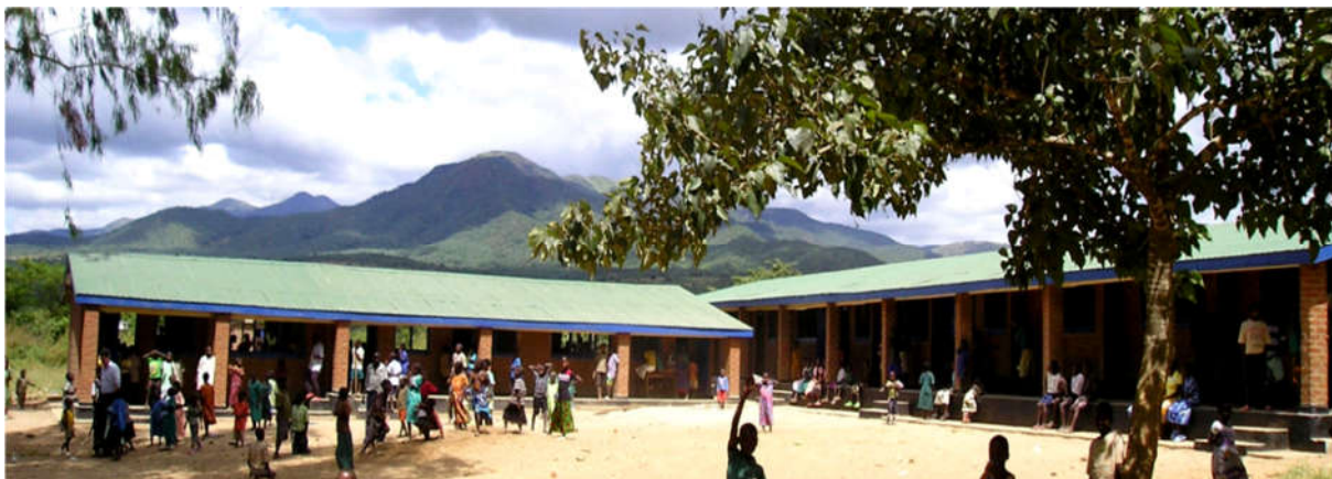
Figure 5: New buildings at local school constructed by Paladin (Africa) Limited
