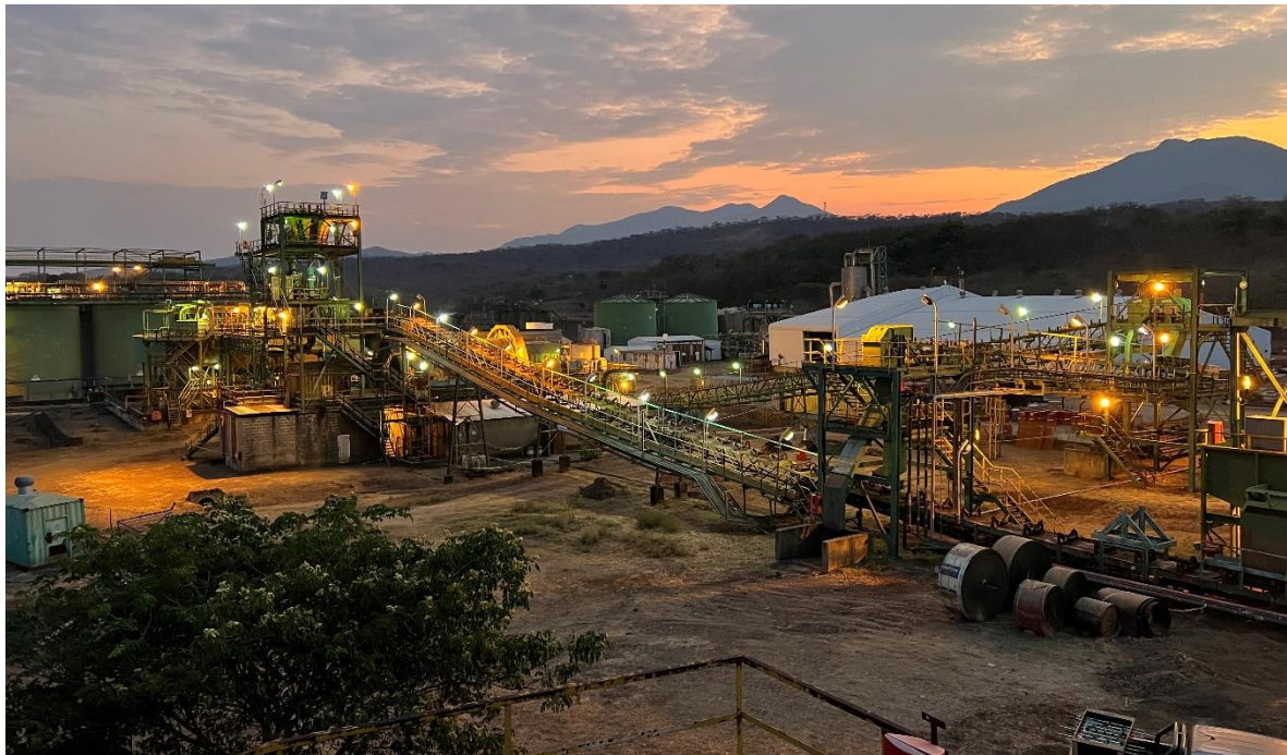
Figure 5: Crushing and grinding plant at Kayelekera
