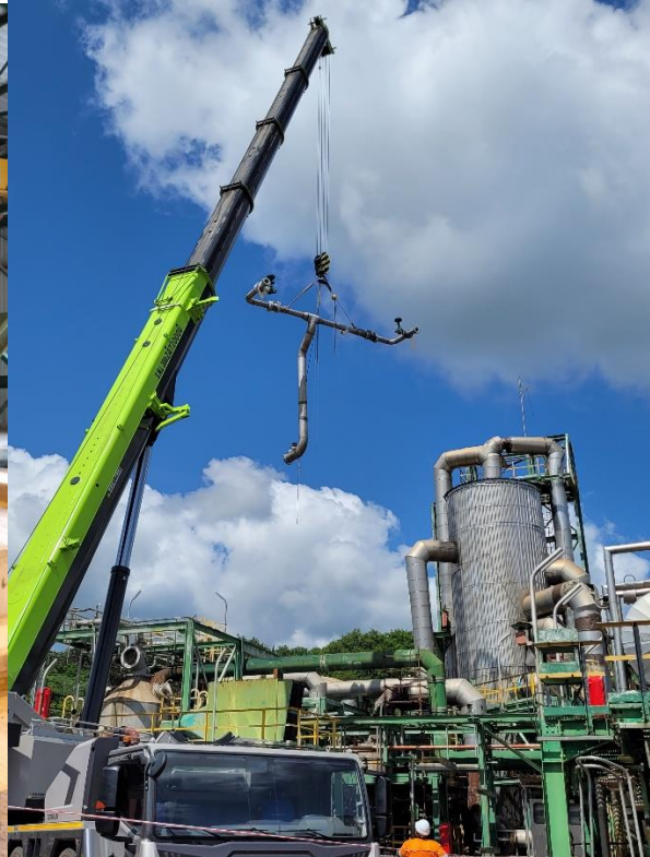
Figure 4: Acid plant refurbishment
