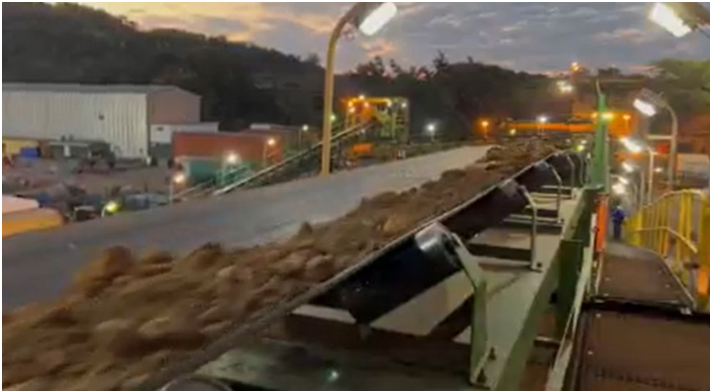
Figure 3: Mill feed conveyor in operation
