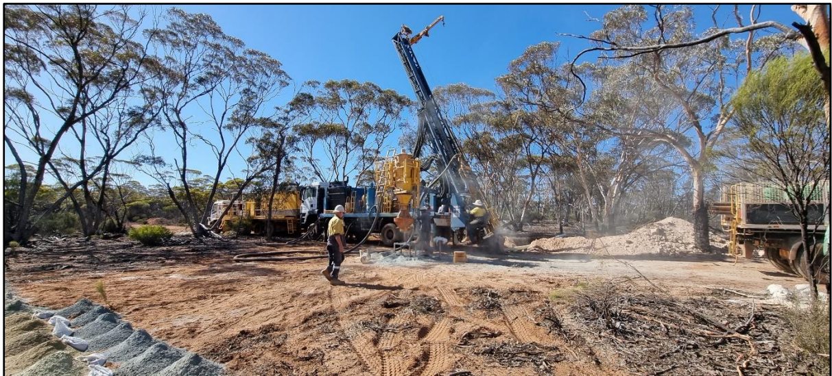
Figure 1 Drill rig on site at Horse Rocks Lithium Project
