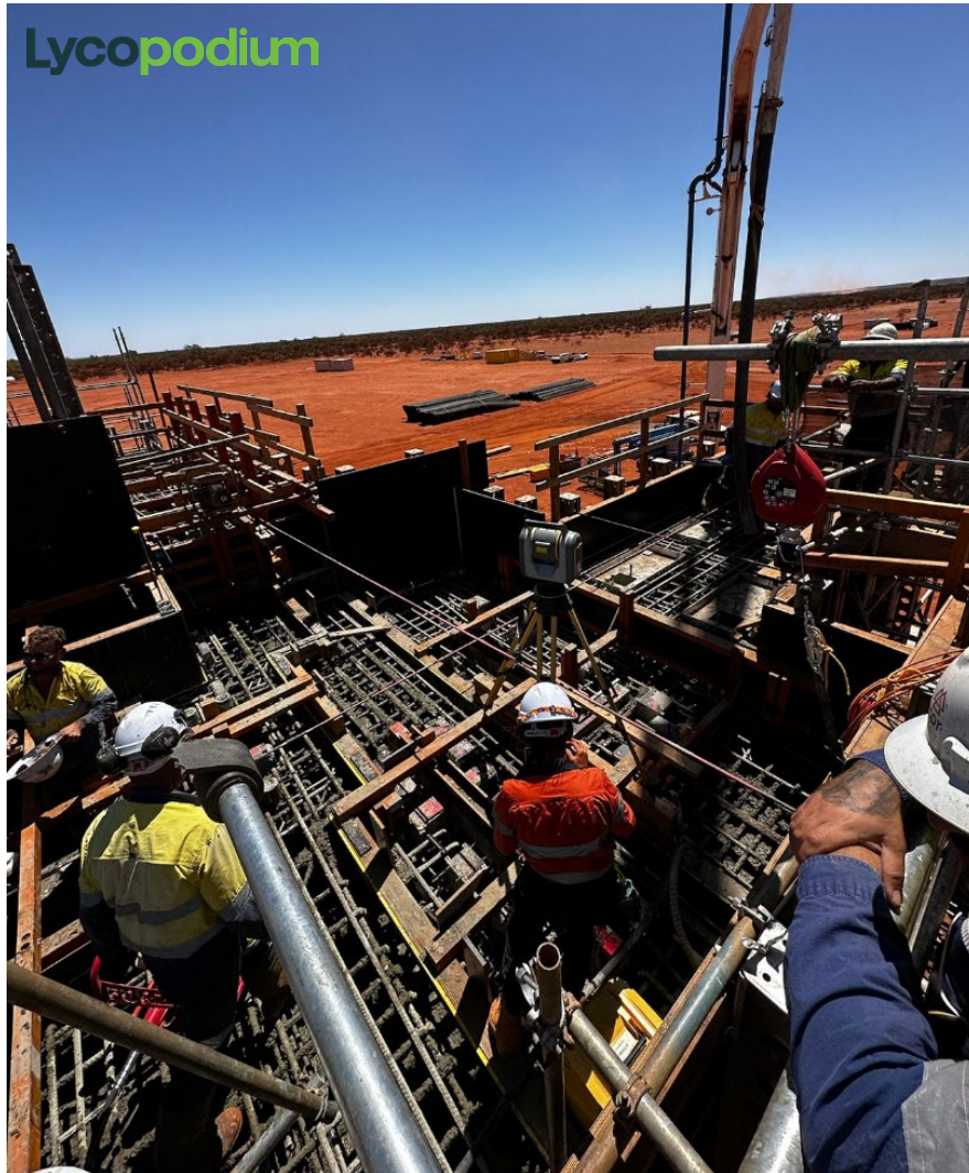
Foundation for the SAG Mill well advanced
