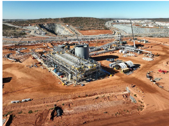
Figure 8: Paste Fill Plant construction well underway
