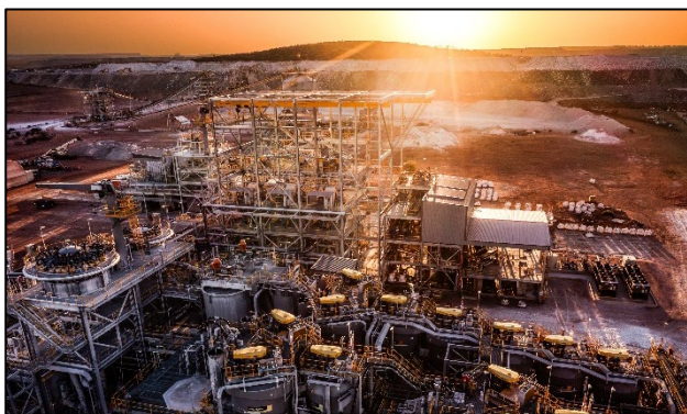
Figure 4: Aerial view of the process plant
