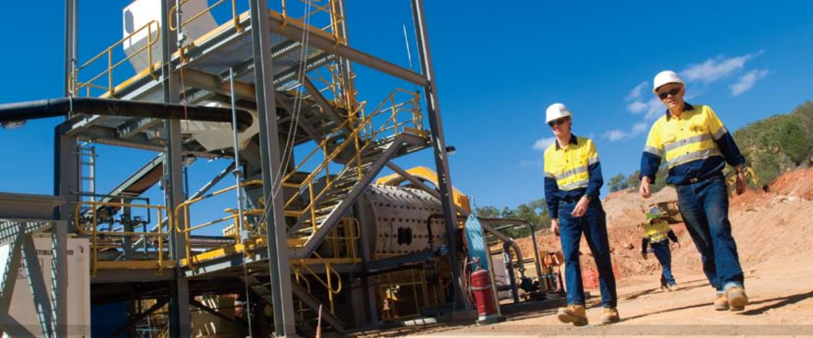
Wolfram Camp Project, Queensland
