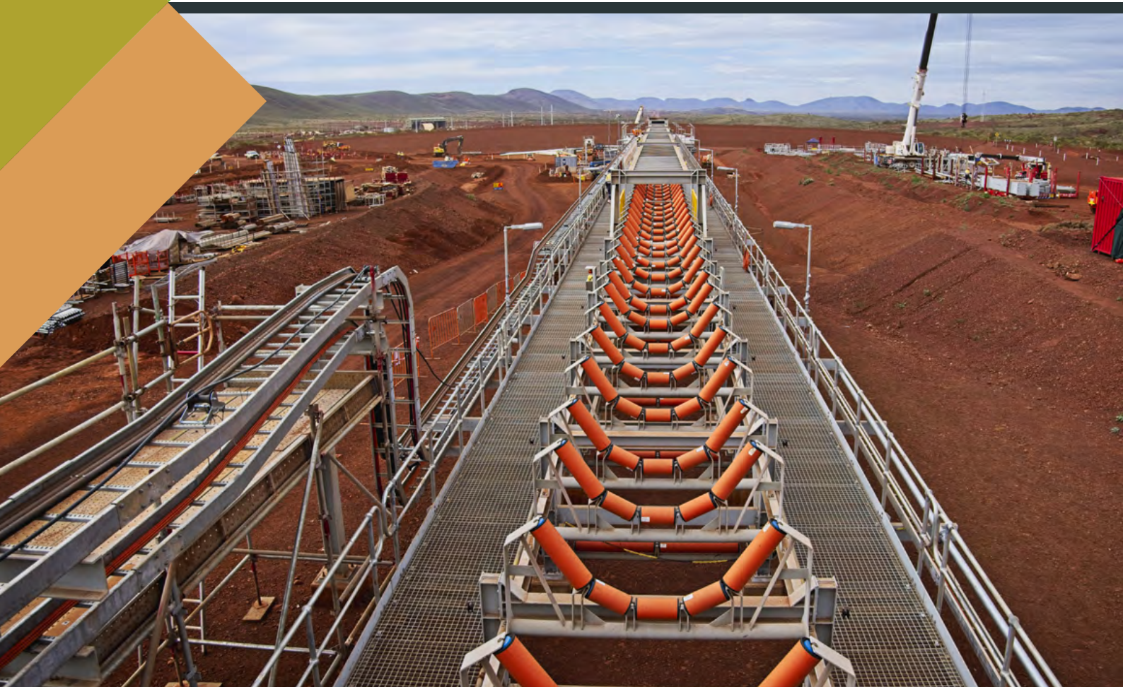
Western Turner Syncline Phase 2 Project, Western Australia
