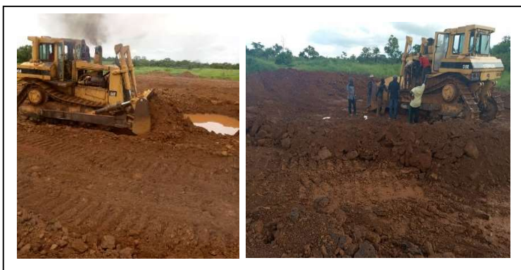
Laterite, iron ore and overburden removal (LHS).
