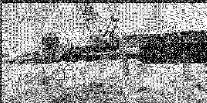
Roe Highway Stage 6 - Bridge construction
