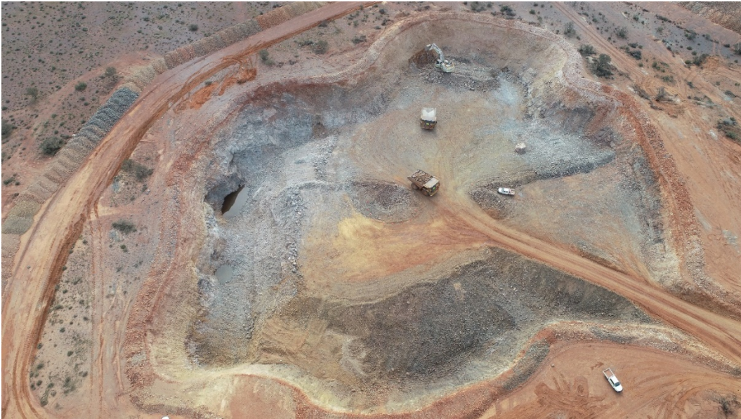
Figure 11: Red Dog Gold Project close to completion of mining
