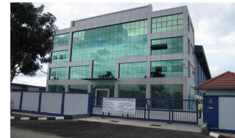
Manufacturing Plant, Kuala Lumpur Malaysia
