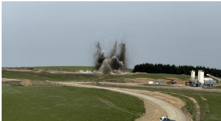
Foundation blasting at Kaiwera Downs
