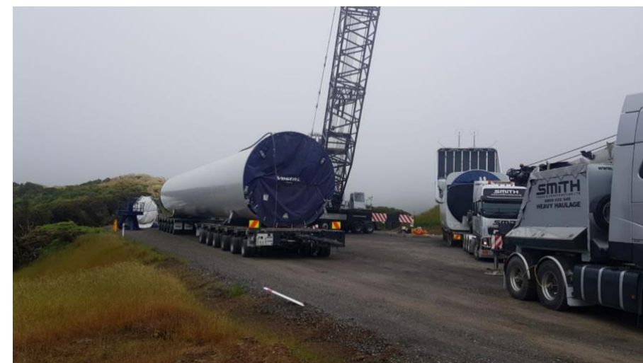
Towers being transported to site for erection
