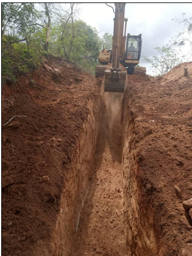
Figure 5 – Trenching begins at the Dragon Target
