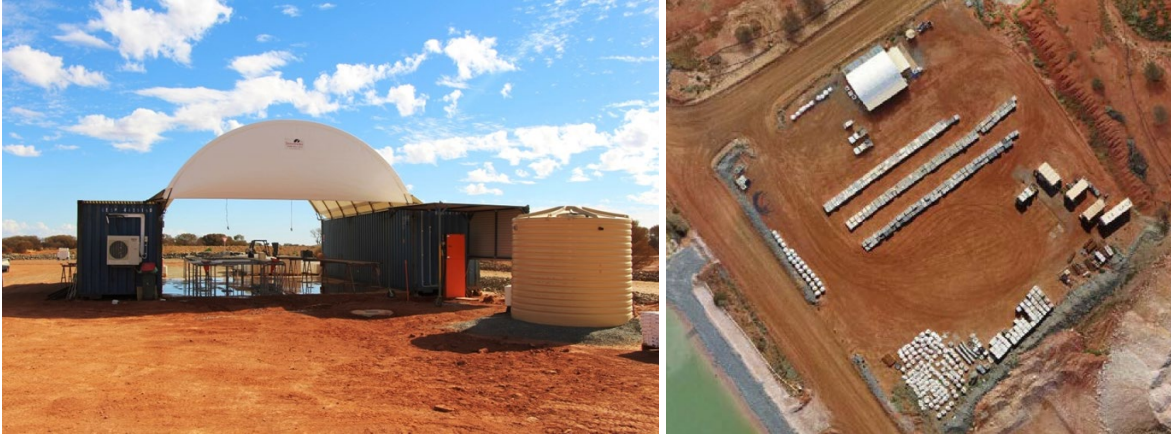
Figure 55 – Andy Well core yard (dome shelter needs to be reinstated).
