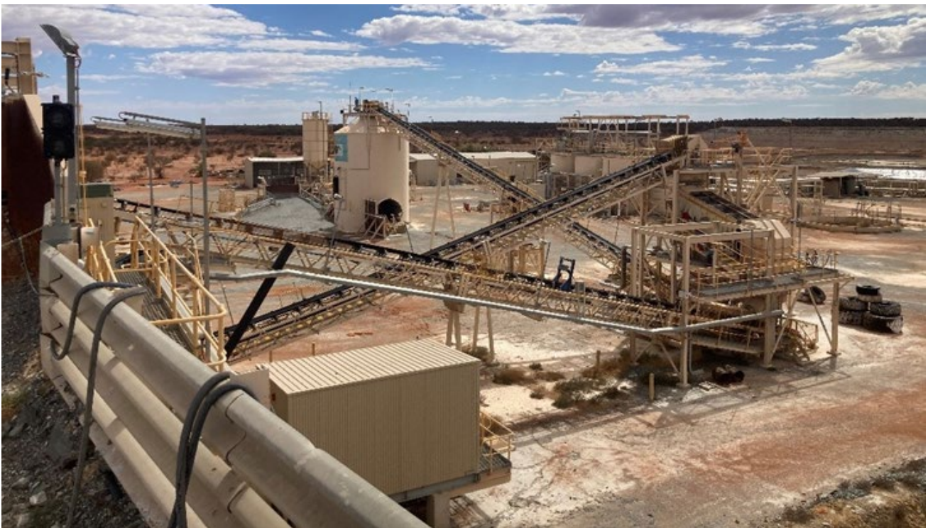
Figure 37 – View of screen deck from ROM feed bin looking north.
