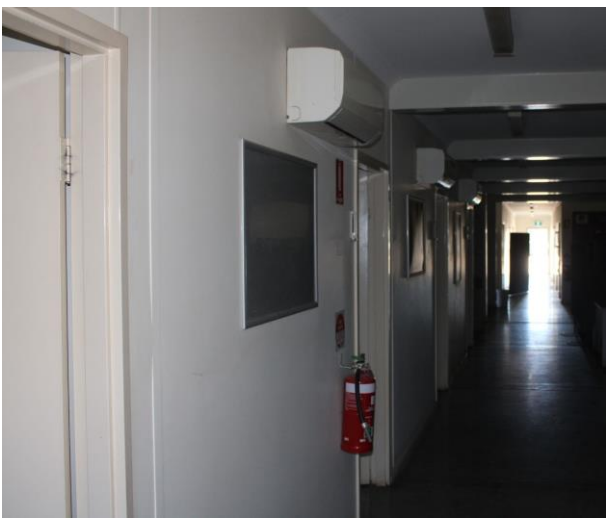
Figure 5: Inside 36.5m x 14.5m office building.
