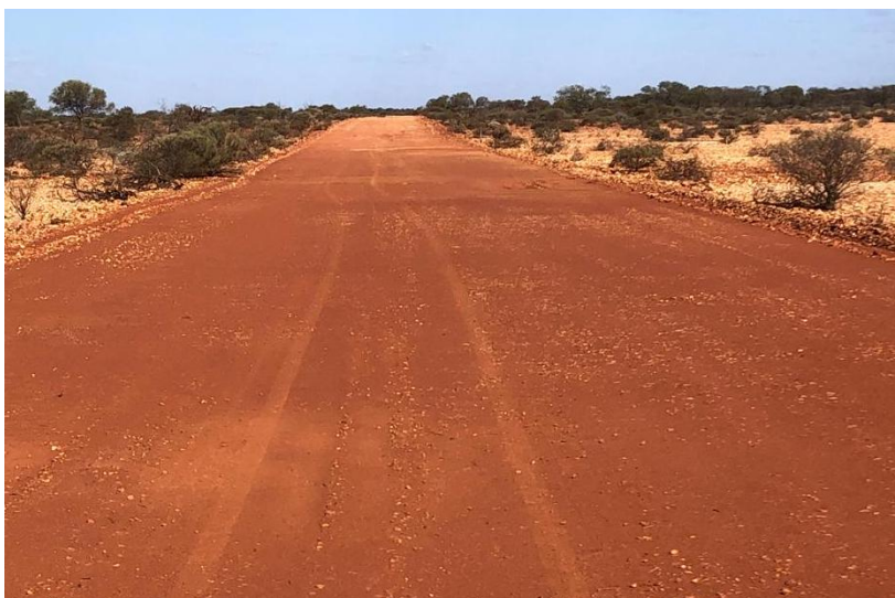
Figure 7: New 20km haul road, November 2024.
