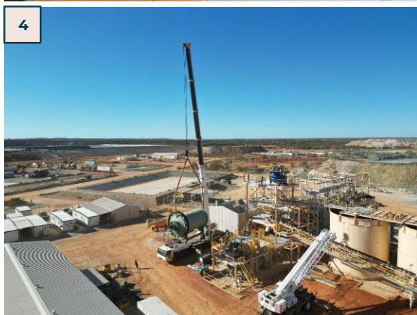
Figure 3: Series showing the 750kW ball mill being lifted into position, March 2025.
