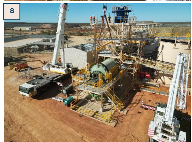
Figure 3: Series showing the 750kW ball mill being lifted into position, March 2025.
