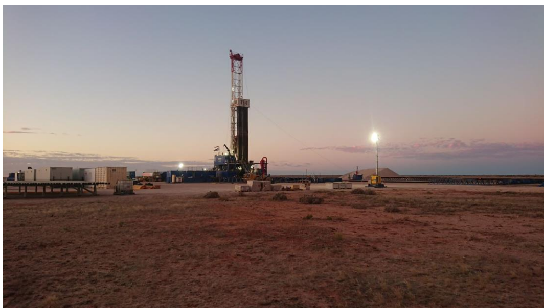
Figure 2: SLR184 rig drilling Odin-1
