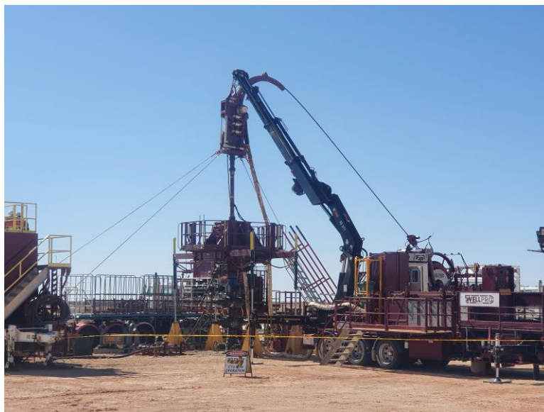
Figure 1: Flow testing operations at Odin-1
