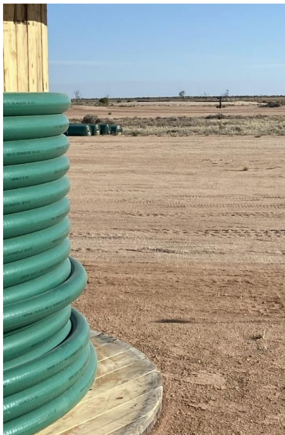
Flowline ready for installation at Odin
