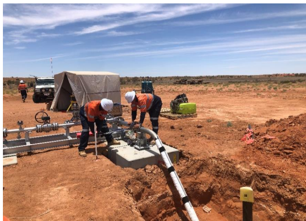
Tie-in of Vali-3
