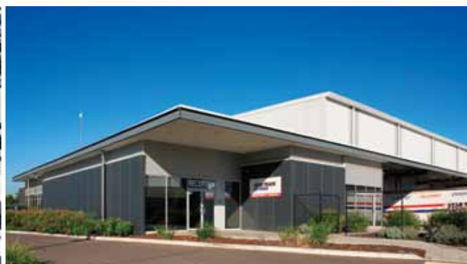
32 SARGENTS ROAD, MINCHINBURY, NSW
