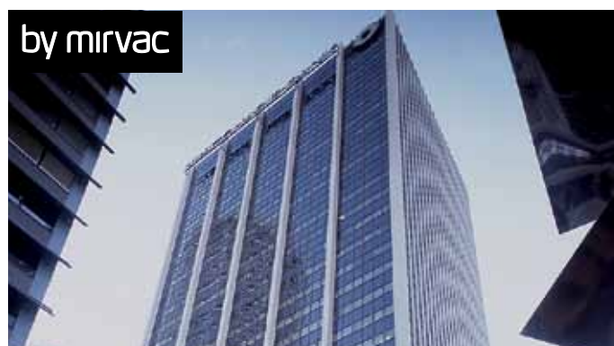
10 - 20 BOND STREET, SYDNEY, NSW IN PROGRESS
