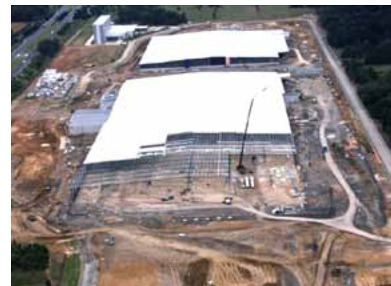
WOOLWORTHS DISTRIBUTION CENTRE, HOXTON PARK, NSW
