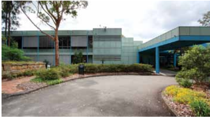
55 COONARA AVENUE, WEST PENNANT HILLS, NSW
