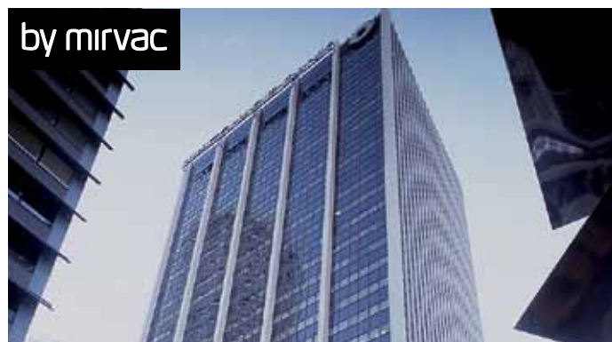
10 - 20 BOND STREET, SYDNEY, NSW IN PROGRESS
