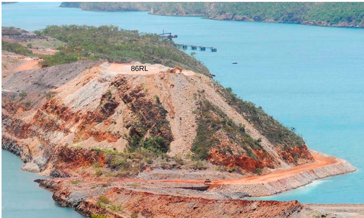
Figure 17 - Blinker Hill mining commences the Main Pit cut back and provides fill material for Main Pit seawall
