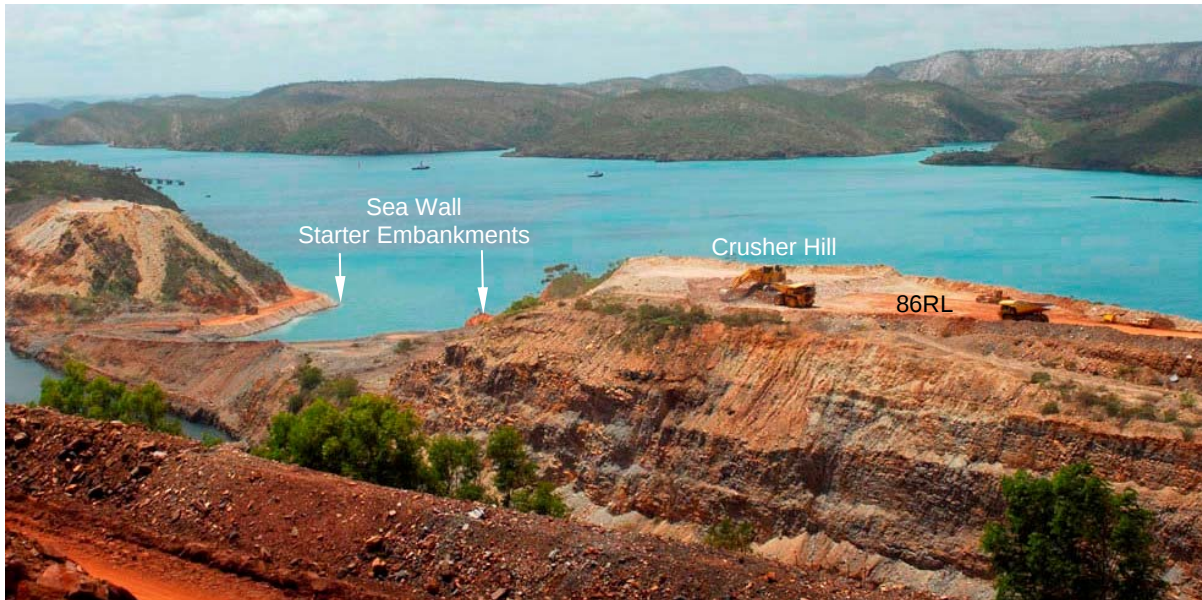
Figure 16 - Crusher Hill mining commences the Main Pit cut back and provides fill for Main Pit seawall
