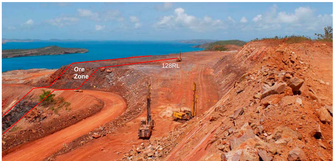
Figure 14 - Main Pit West – December 2007
