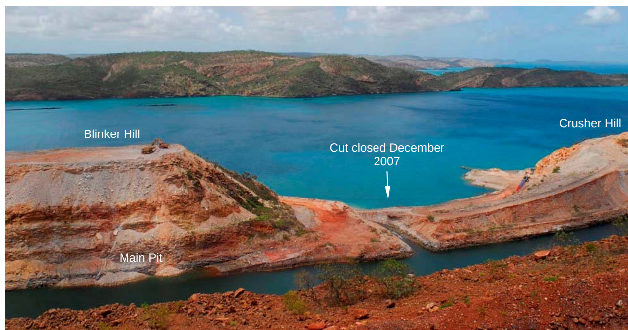
Figure 15 – Seawall access ramp placed across tidal channel into Main Pit established in December 2007
