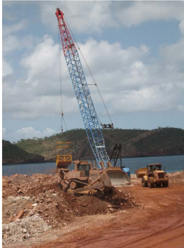
Figure 18 – Main Pit seawall construction commencing December 2007
