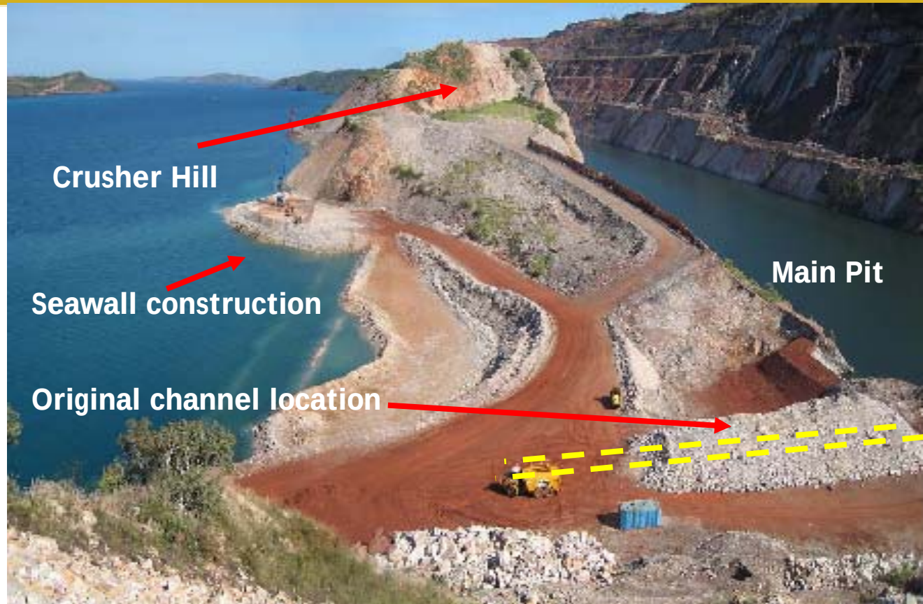
Main Pit - March 2008
