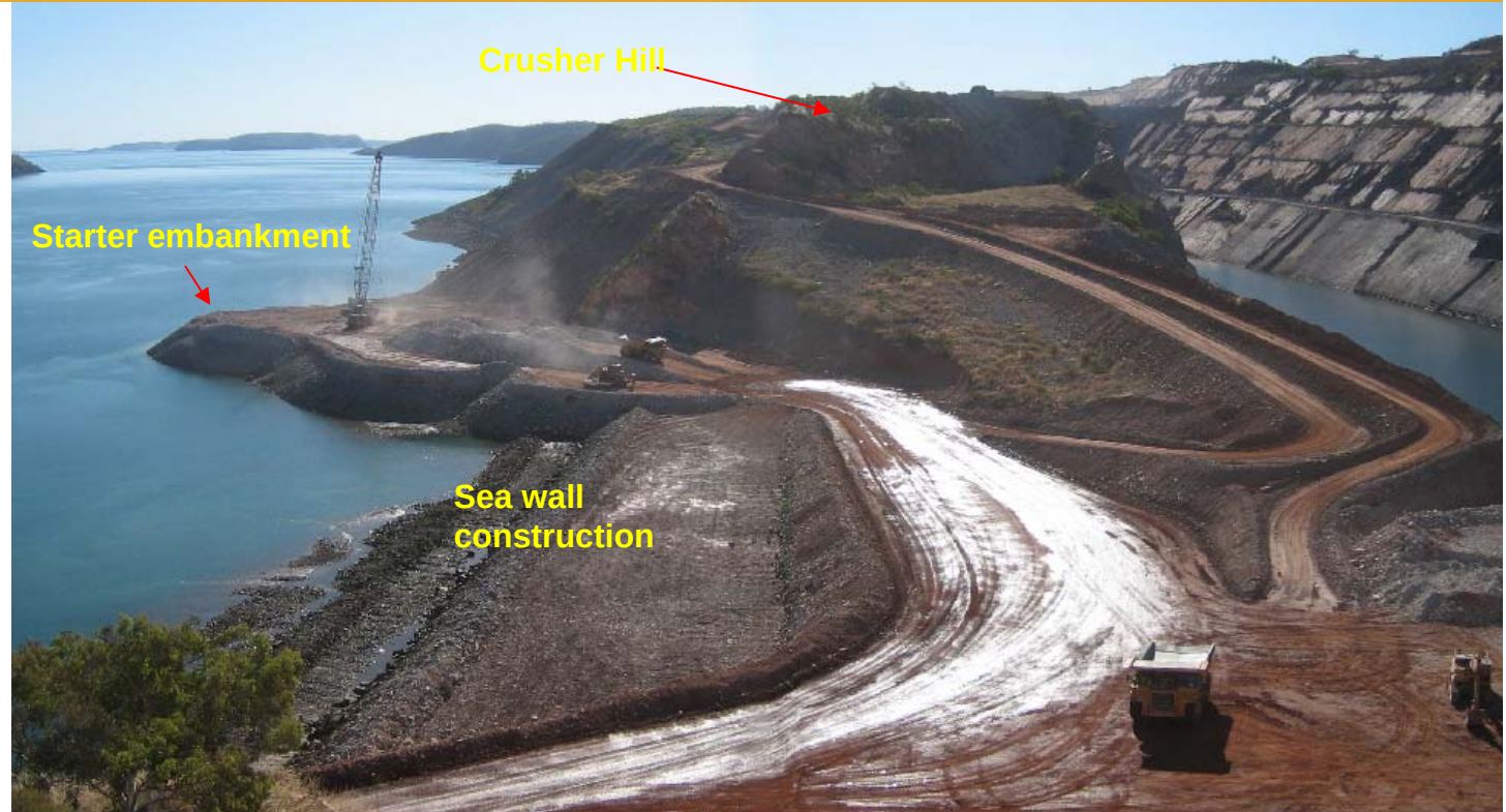
Main Pit seawall construction - June 2008
