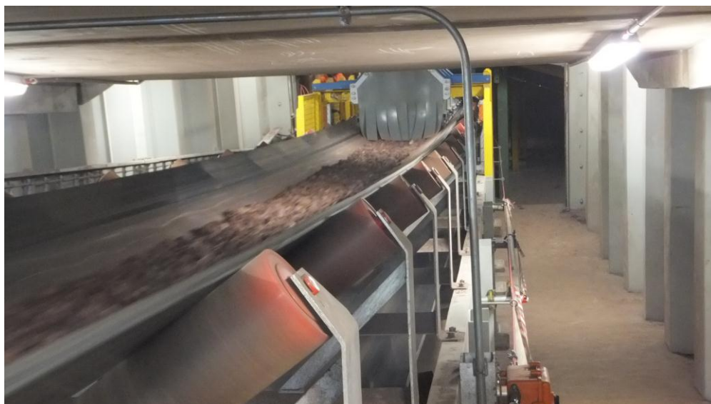
Figure 4 – The new unloader in action.
