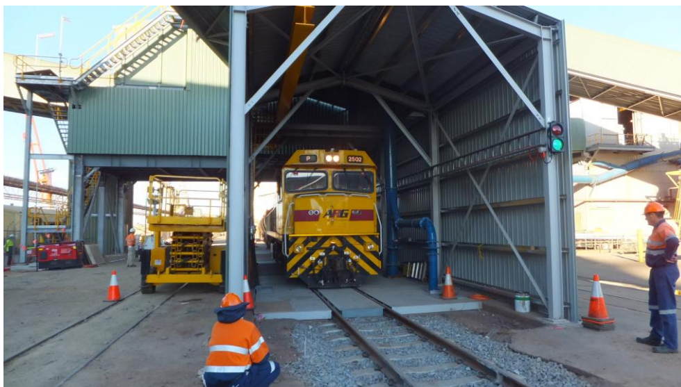
Figure 3 – The new train unloader receives its first train.
