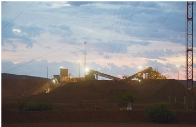
Extension Hill processing
