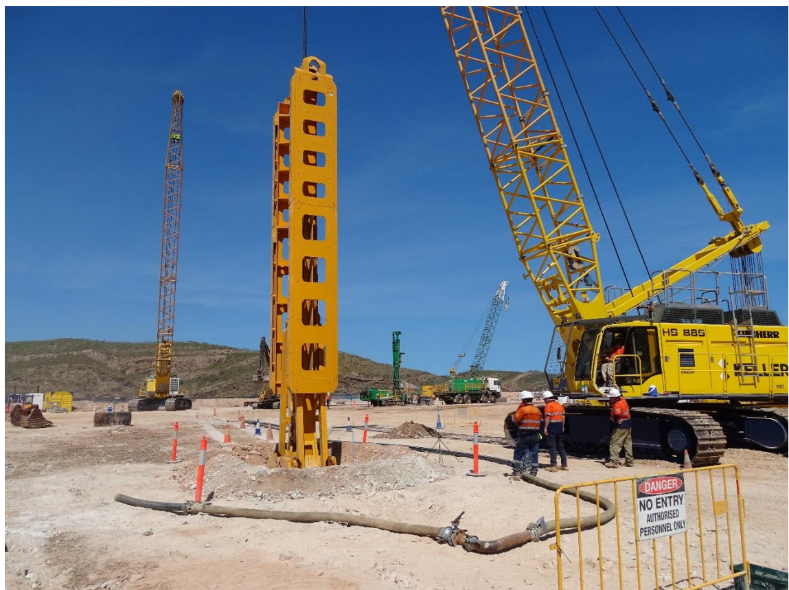
Figure 7: Pilot seepage barrier panel excavation – 28 September 2017
