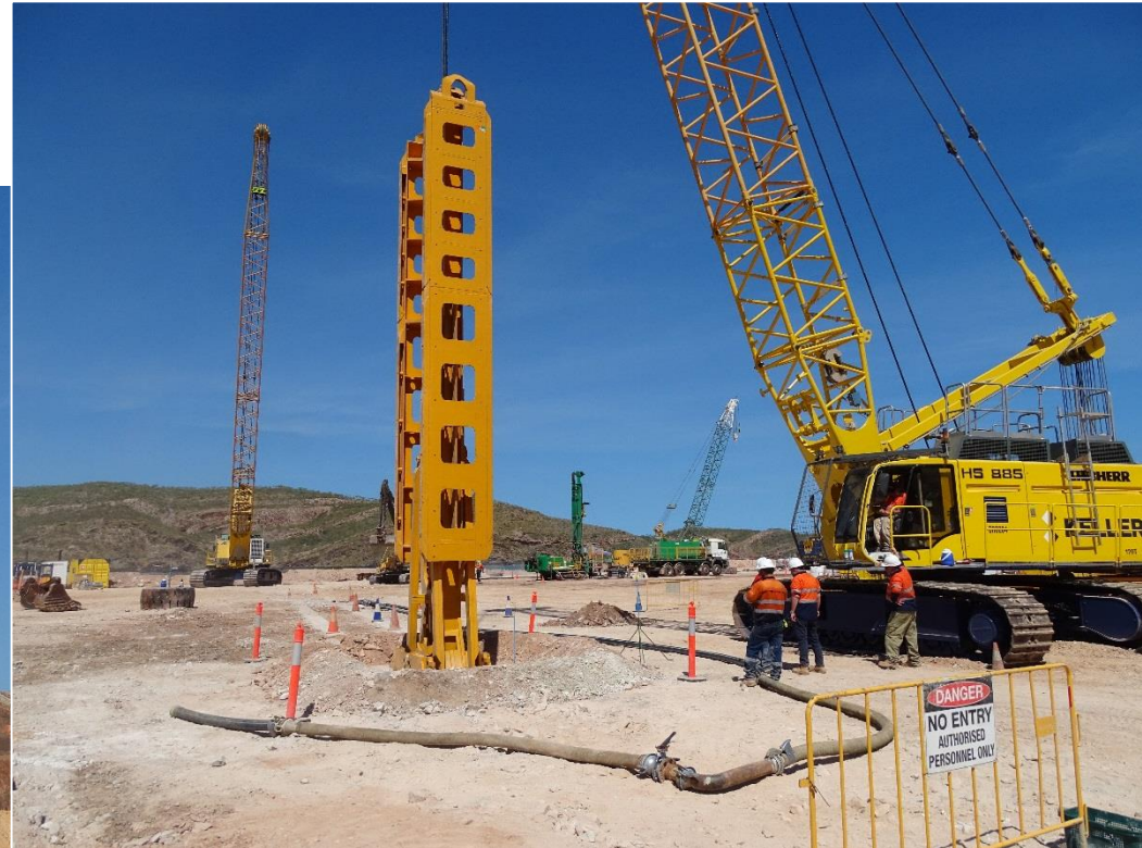
Excavation of pilot seepage barrier panel, September 2017.
