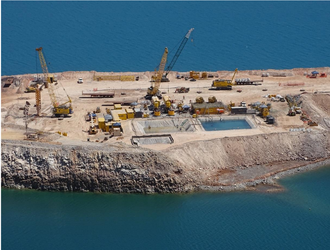
Seepage barrier construction preparations, showing excavators, bentonite plant and ponds, September 2017.
