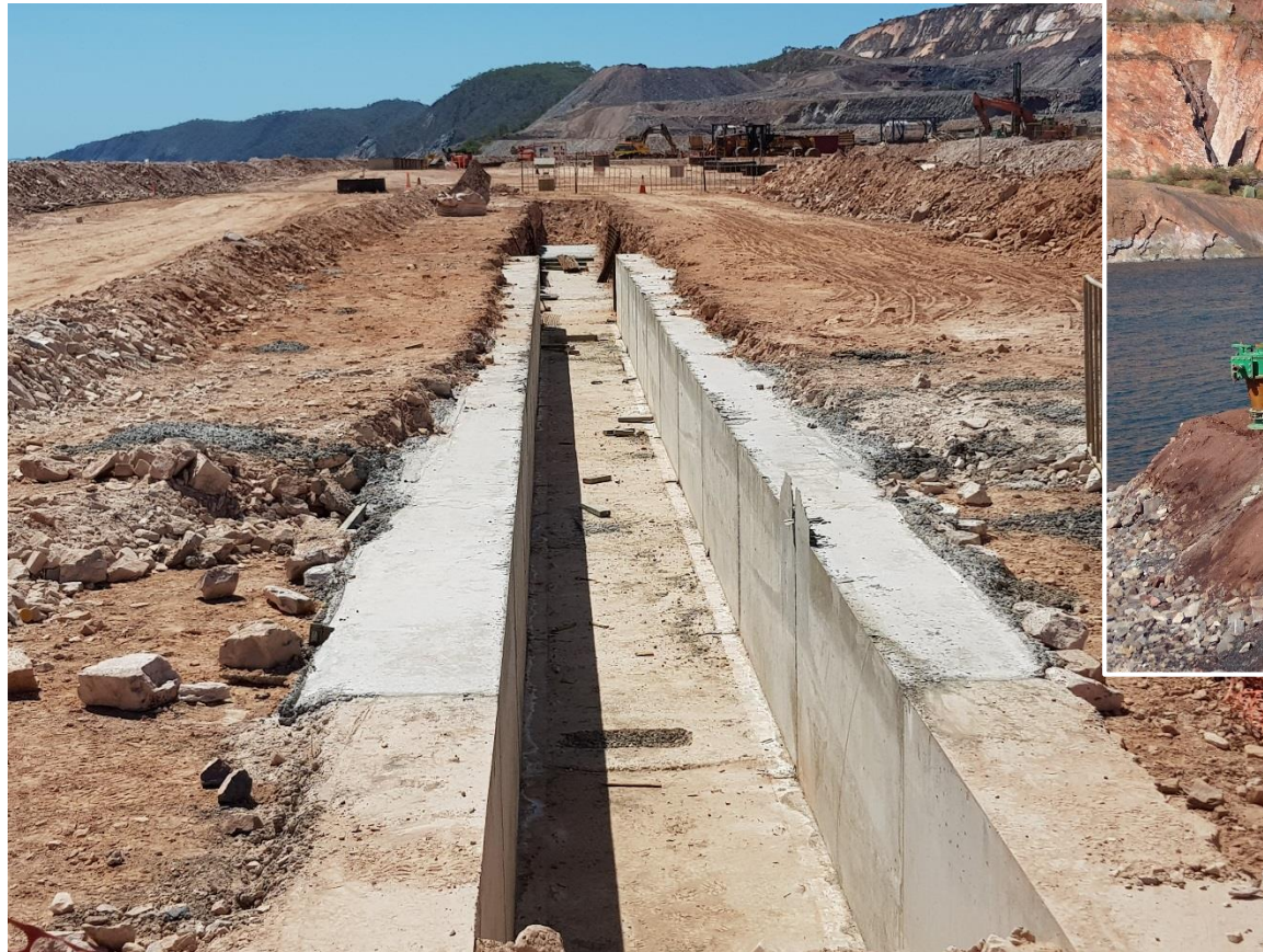
Seepage barrier guide wall construction, October 2017.
