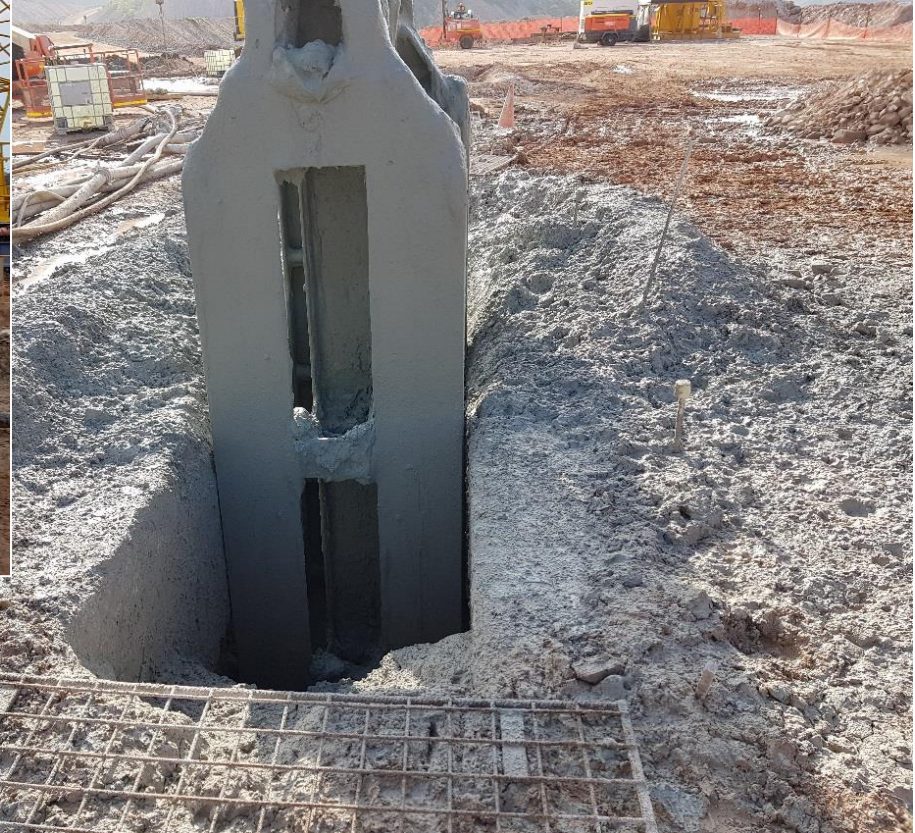
Grabber excavation of Panel 050 - December 2017
