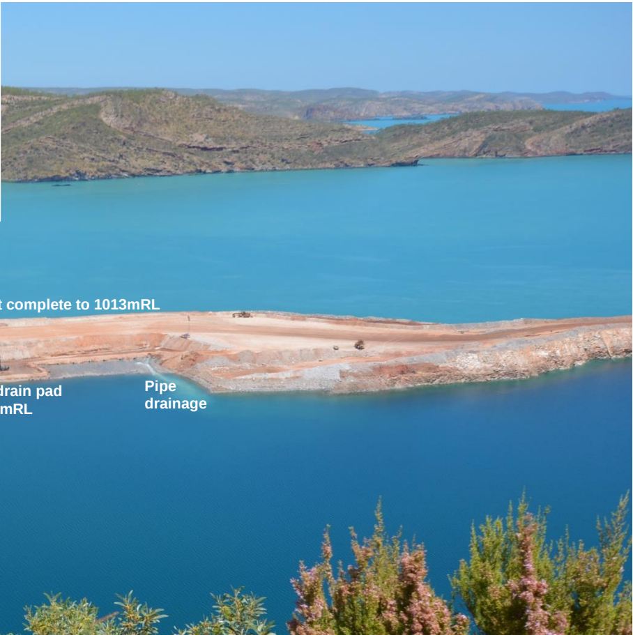
Completed embankment, September 2017
