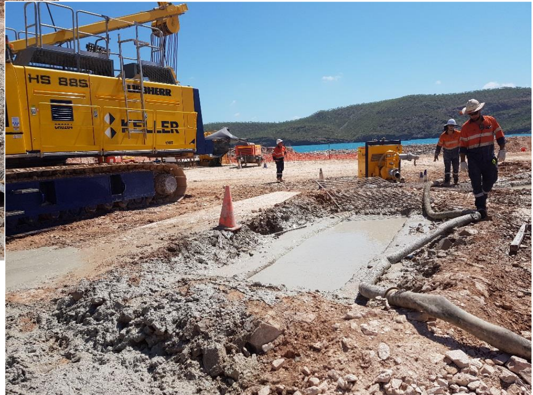
Completed Panel 030 – December 2017
