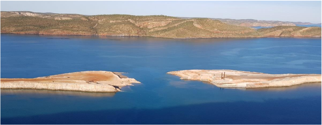
Starter embankment construction in July 2017
