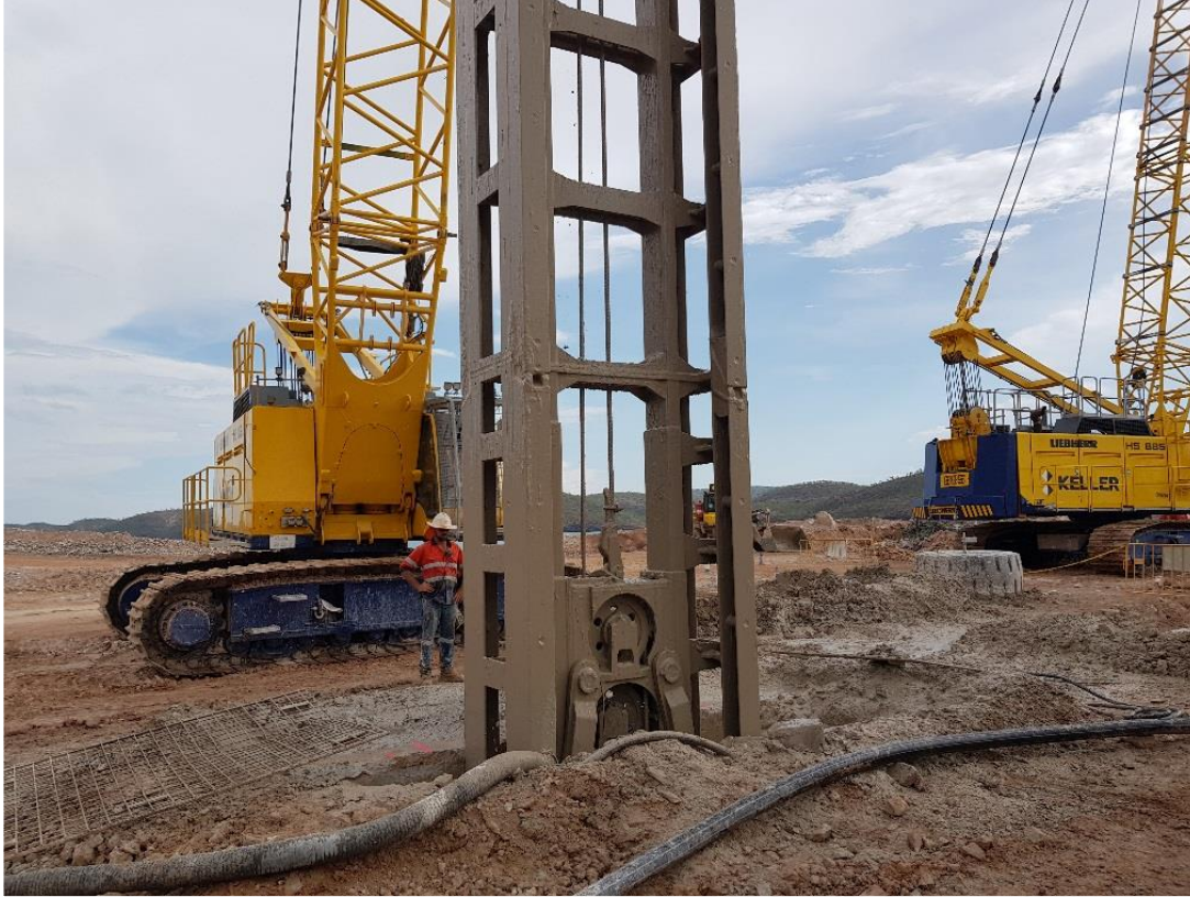
Grabber excavation of Panel 016 - December 2017
