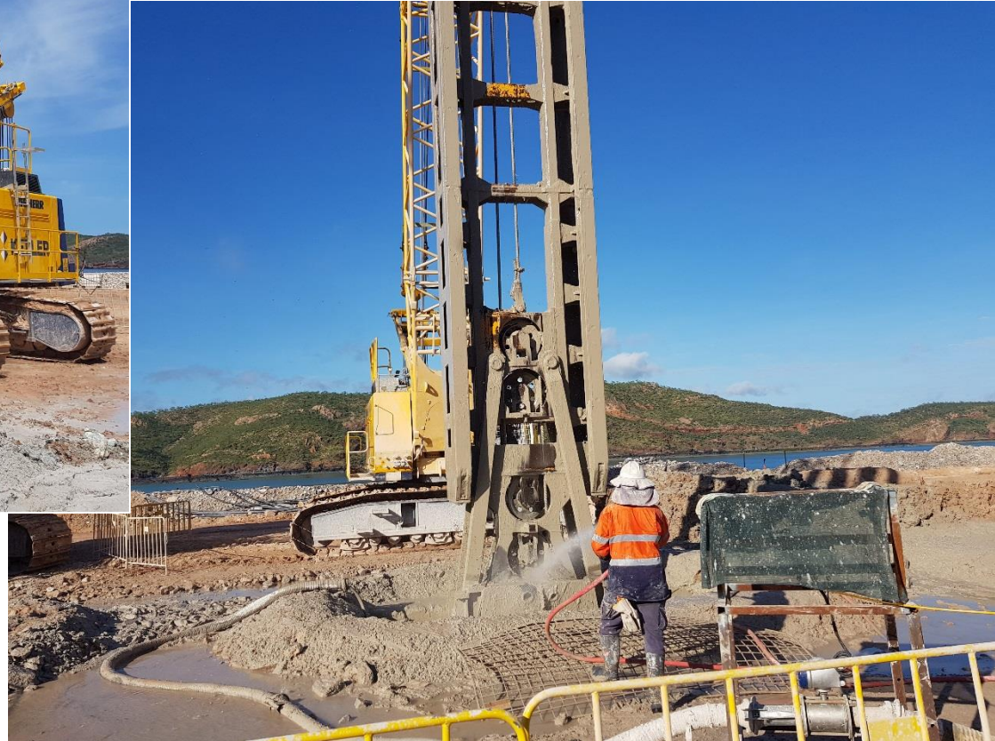
Panel excavation, March 2018
