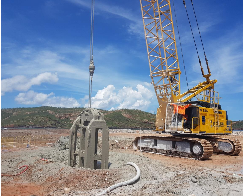
Grabber excavating seepage barrier panel March 2018
