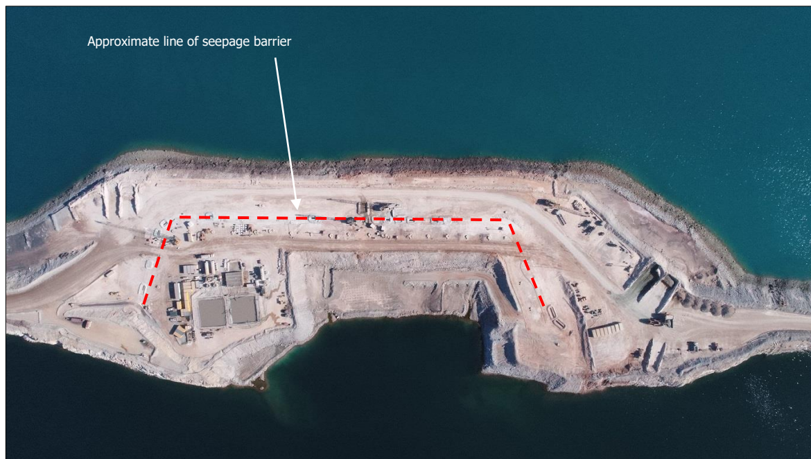
Figure 2: Aerial view of seawall embankment – end June 2018
