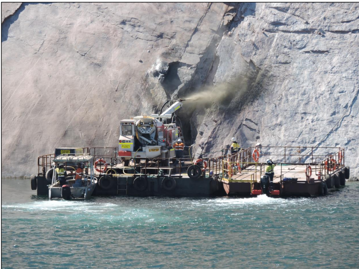
Figure 7: Shotcreting of Main Pit Footwall – July 2018
