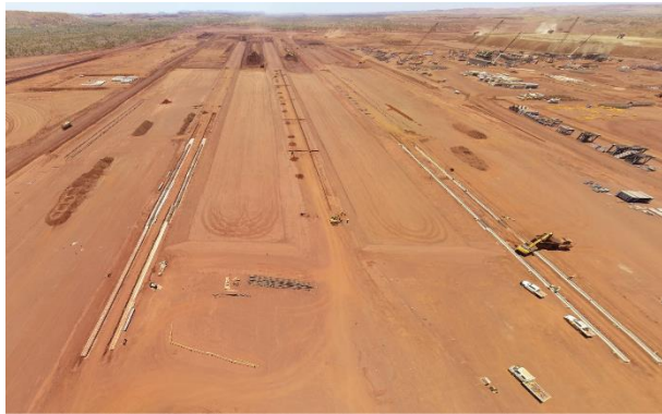
Stacker works and stockyard earthworks
