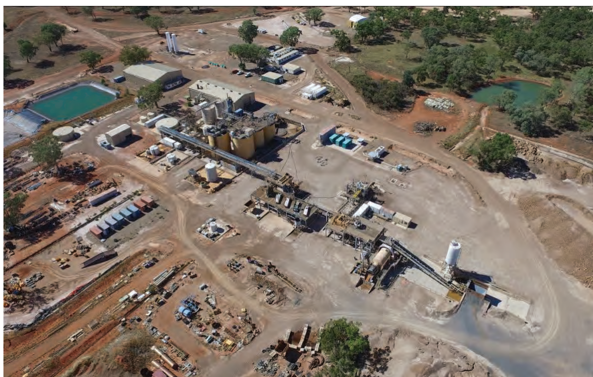
Figure 17-1: Aerial view of the Wonawinta plant.
