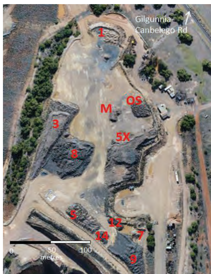
Figure 14-7: ROM Pad Stockpiles.
