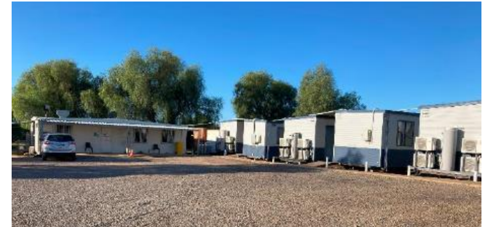
Existing Camp located at Mt Boppy
