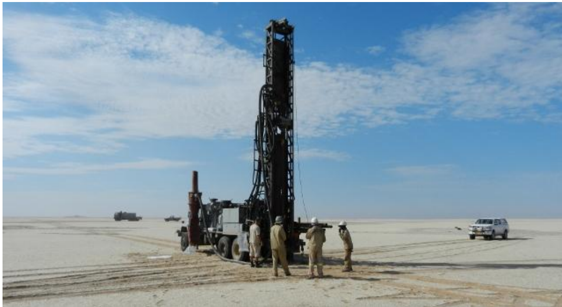
Figure 1 – Drilling underway at Mile 72.
