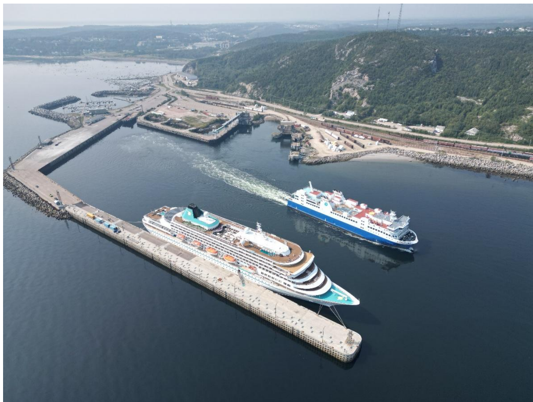
Figure 4: Port of Baie-Comeau
