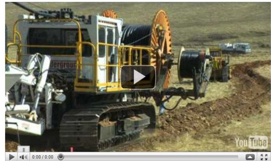
Underground Services ploughing technology installing 315mm pipeline
